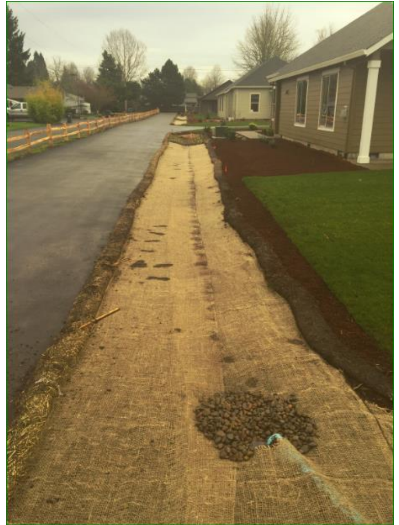
Drive & LIDA swale along entire length
